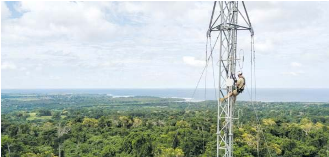
Army telecommunications riggers Cpl Cameron Poole installs a very high frequency radio microwave antenna onto Erakor cellular tower during Phase 2 of the Vanuatu Government national emergency radio network. Photo: Cpl Olivia Cameron
